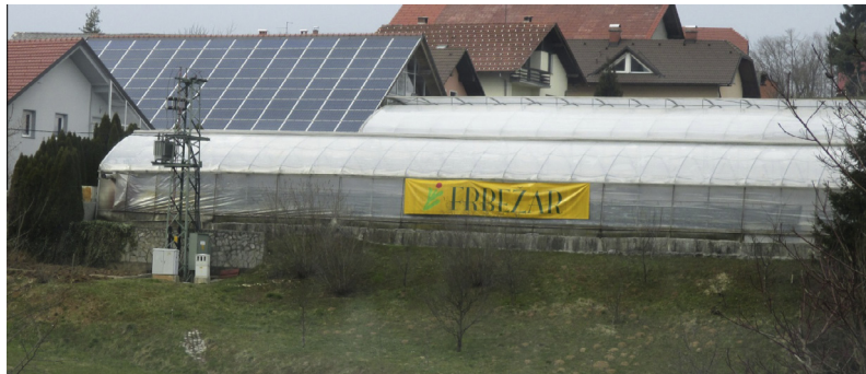
Fig. 7. The photovoltaic solar power plant installed on the roof of the administrative building of the "Frbežar" nursery garden.
