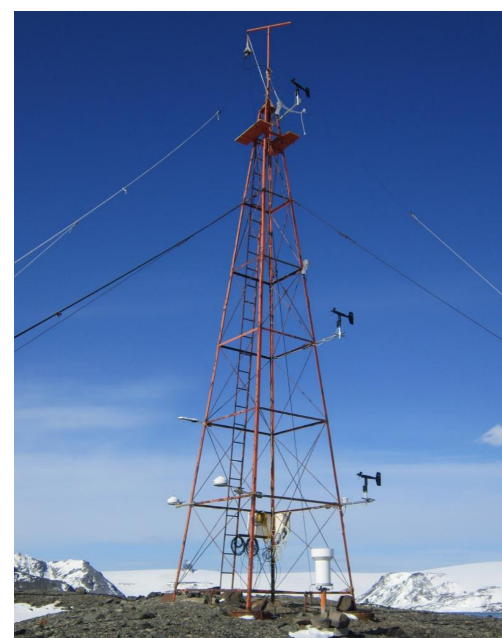
Figure 2: East view of the 12 meter instrumented South Tower.
